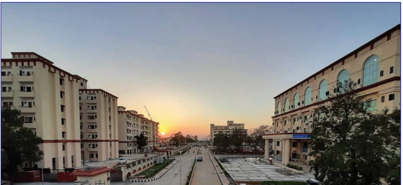
NTPC Medical College & Hospital Project, Sundargarh, Odisha
