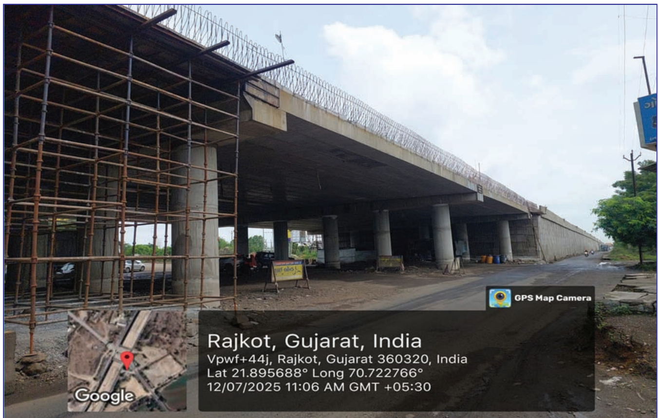
NHAI, Rajkot Flyover work in Progress
